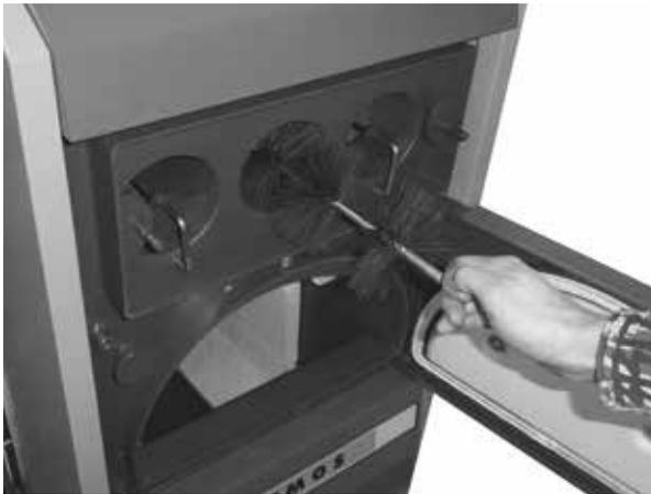
Cleaning of (tubes) exchanger with inserted the brush (by boiler D20P, D30P, D40P, D50P)
