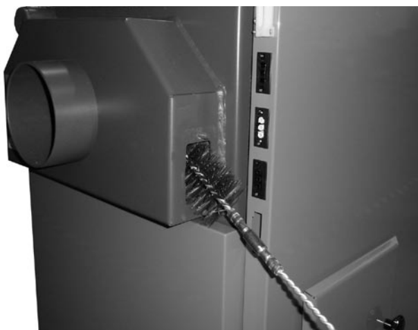
Sample cleaning of the smoke channel. It is performed after cleaning of the tube plate in the combustion chamber of the boiler
