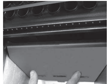
Pict. 14: Lift the fire shield
